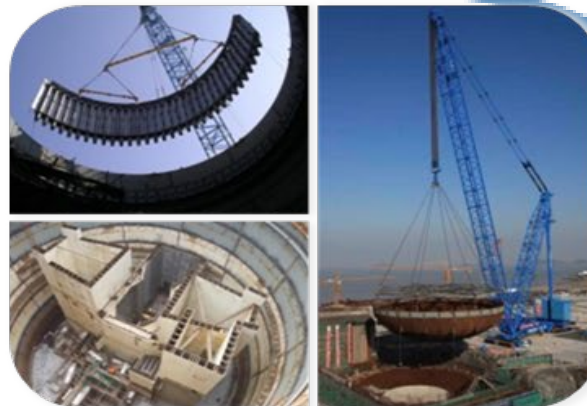
On-site module assembly
