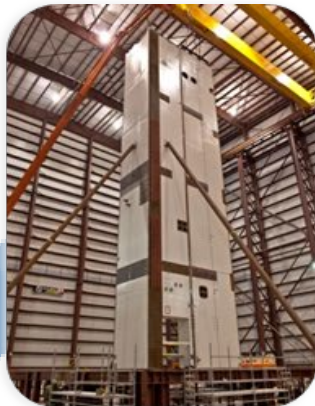
Factory production of modules
