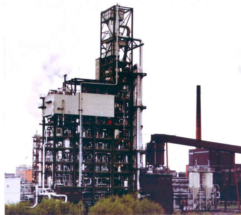
HTW Syngas Plant, Oulu/Finland
