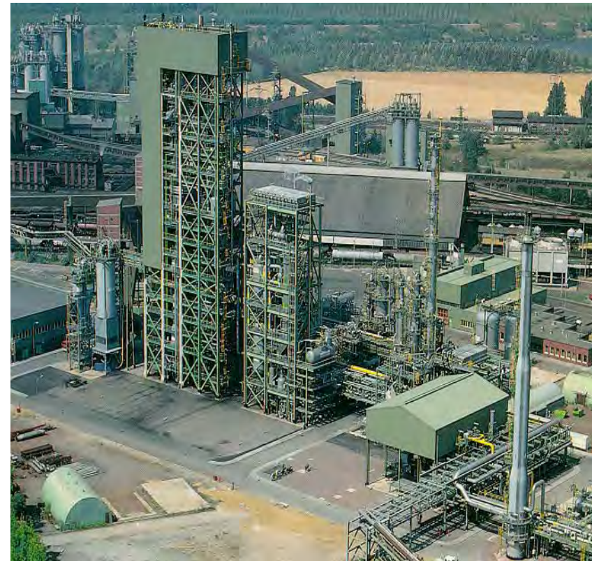
HTW Demonstration Plant Berrenrath, Germany Production Rates: 300 t /d methanol
