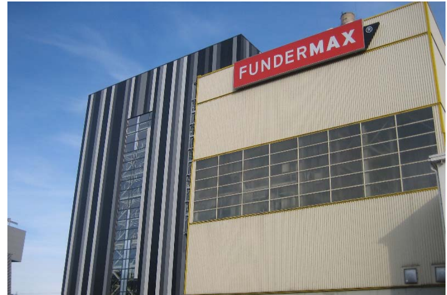
Power plant FunderMAX, St. Veit
