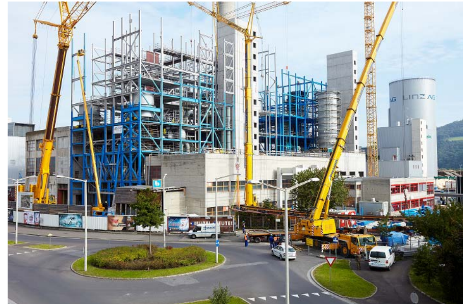
Power plant construction, Industrial area, Linz
