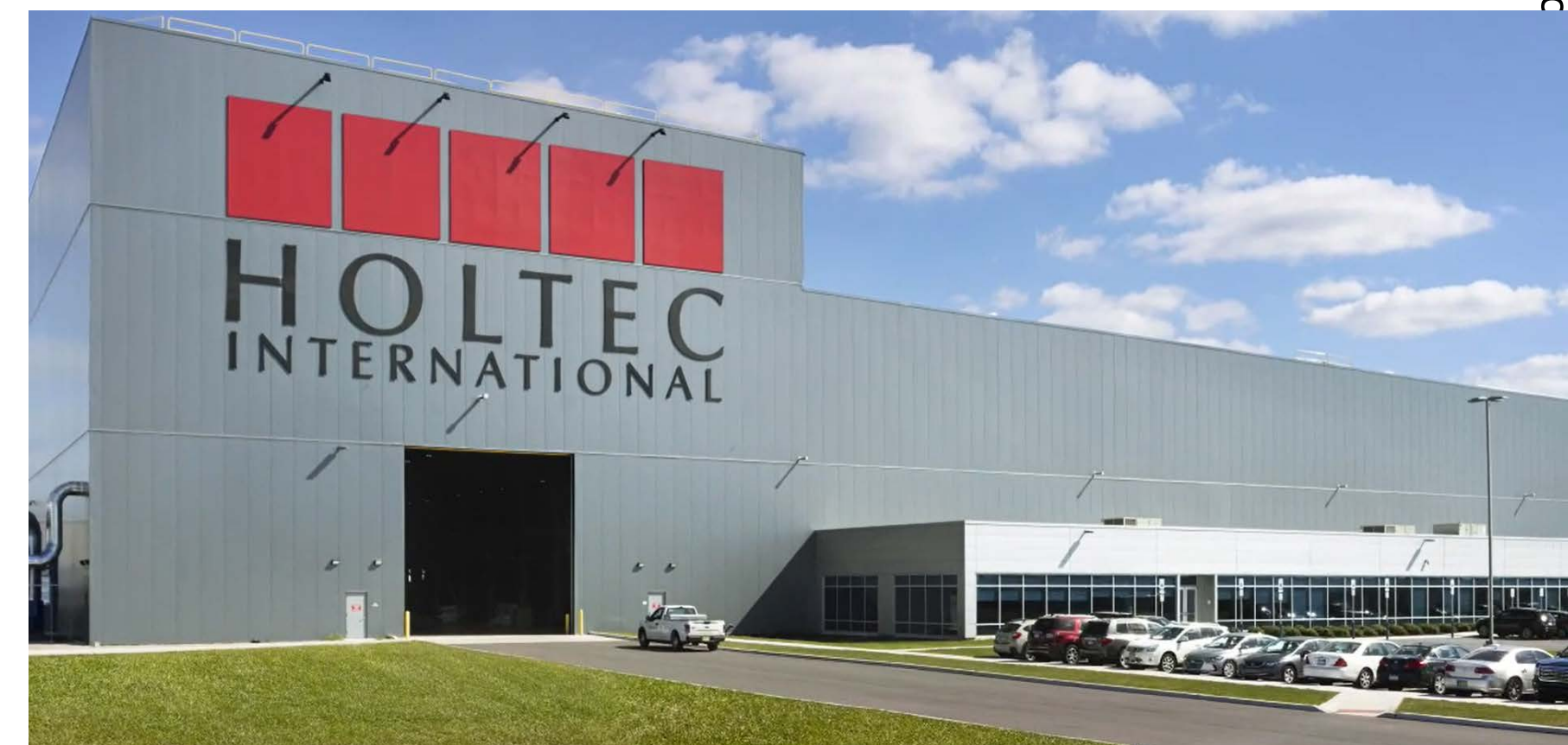
Holtec's Advanced Manufacturing Division (AMD) Designed and Constructed for Fabrication of SMR-160
