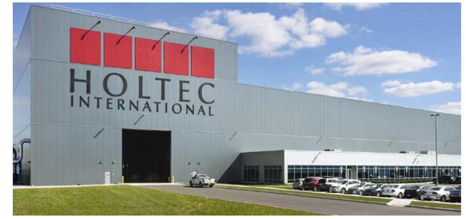
Holtec's Advanced Manufacturing Division
