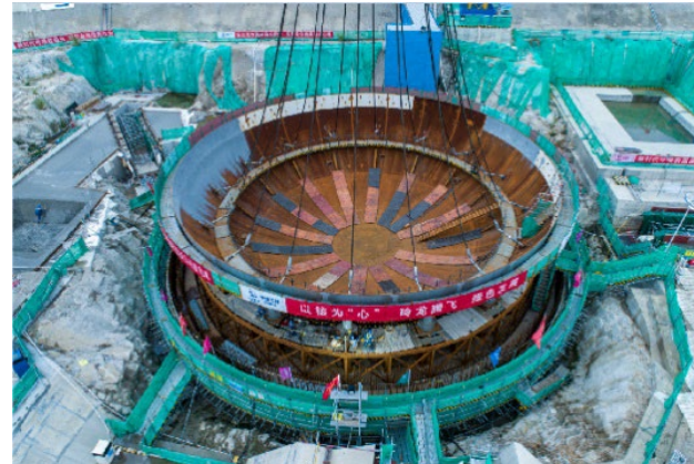
CV Bottom Head Positioned October 24, 2021
