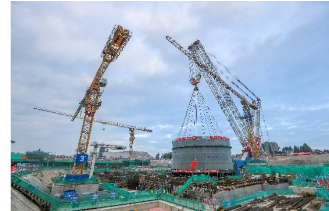
Hoisting of the Lower Cylinder of the Containment Vessel February 26, 2022
