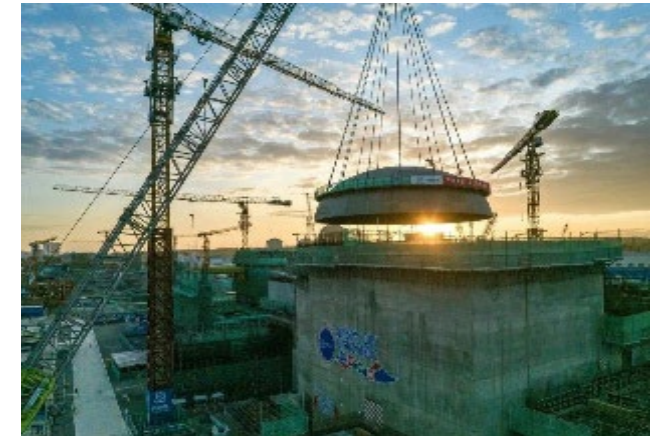
Hoisting of the CV Doom November 3, 2023
