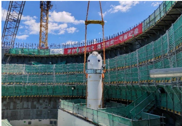
Hoisting of the Pressurizer July 6, 2023
