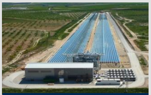
Concentrated Solar Power
