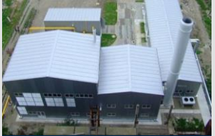
Embedded Co/Tri Generation
