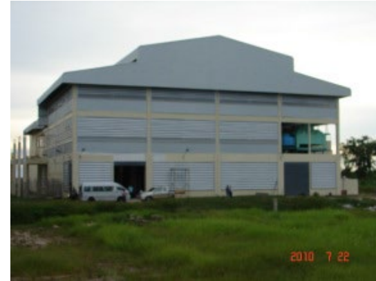
1000 kW Grid connected – Thailand
