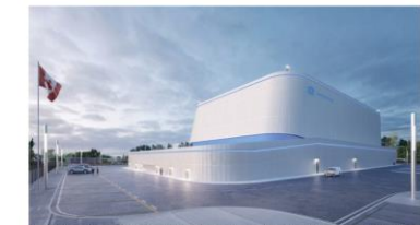
An artist's rendition of a GE Hitachi BWRX-300 nuclear unit. The BWRX-300 is a 300-MW boiling water reactor (BWR) that derives from the Gen III+ 1,520-MW ESBWR, which the Nuclear Regulatory Commission certified in 2014. Courtesy: GEH
